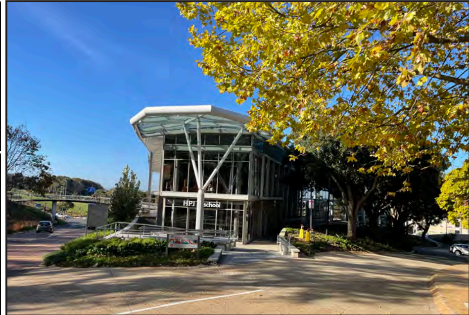
Image: View of the corner entrance of the building from the south-west.
