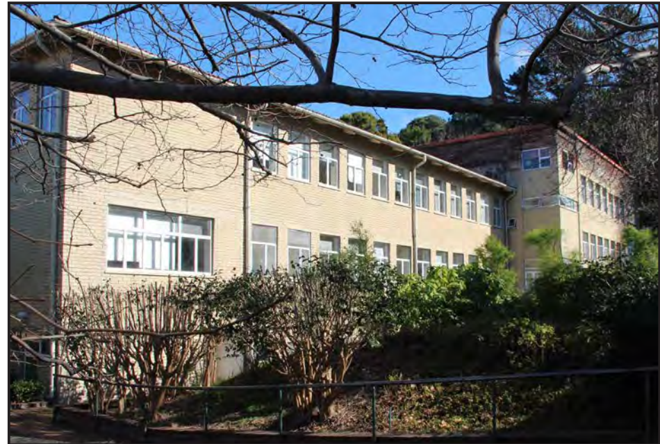
Image: North facade of the building.
