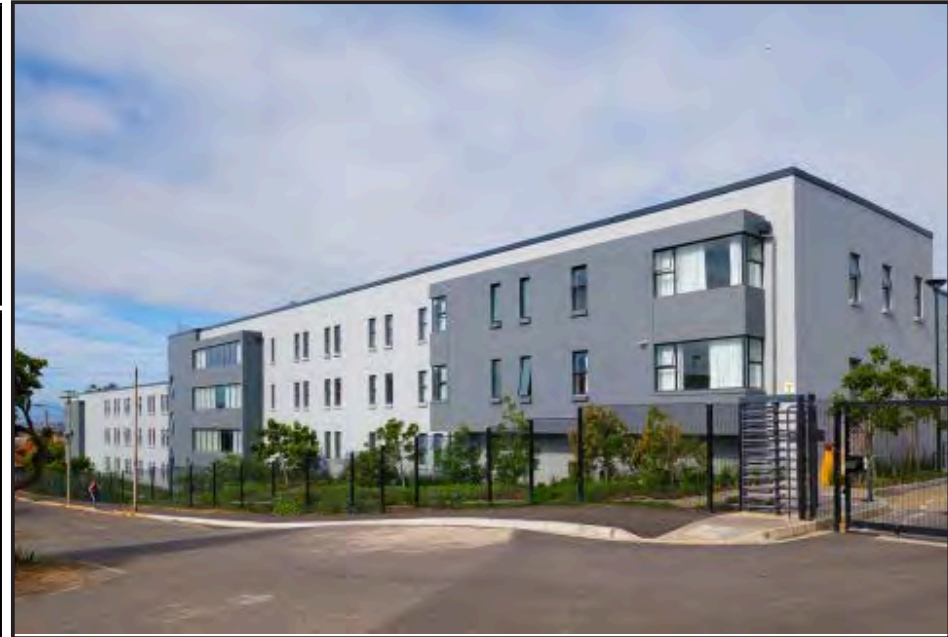
Image: View of the north-facing elevation of Avenue Residence (source: Jakupa Architects &amp; Urban Designers).
