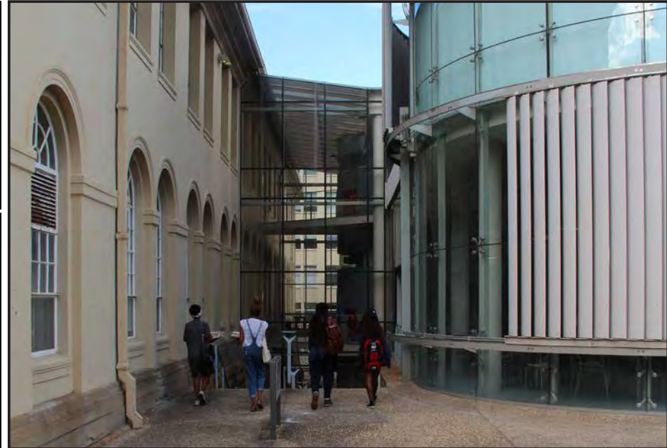
Image: Junction between the Wolfson Pavilion and Wernher-Beit North.
