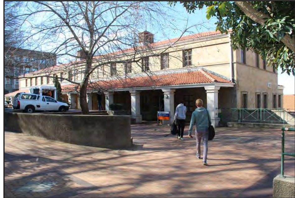
Image: Western approach, facing towards the building.
