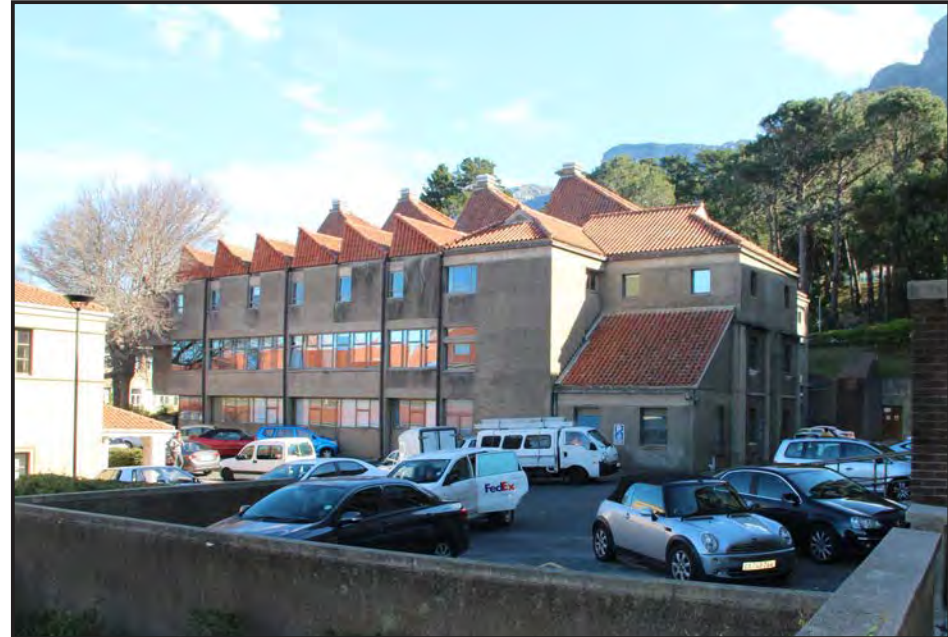
Image: East facade of the building.
