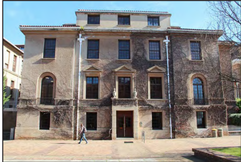
Image: Entrance of the Jaggars Library Building off University Avenue/Jammie Plaza.
