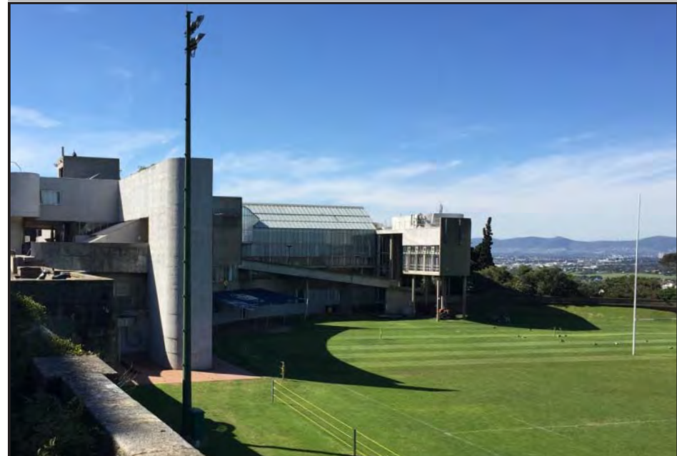
Image: View looking northwards from Rugby Road.
