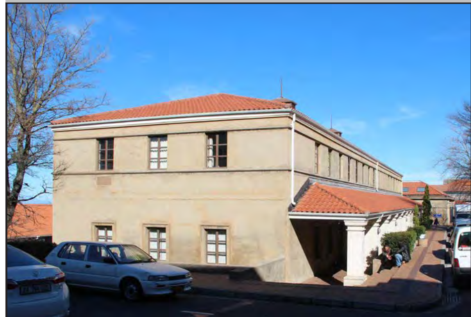
Image: North facade of the building.
